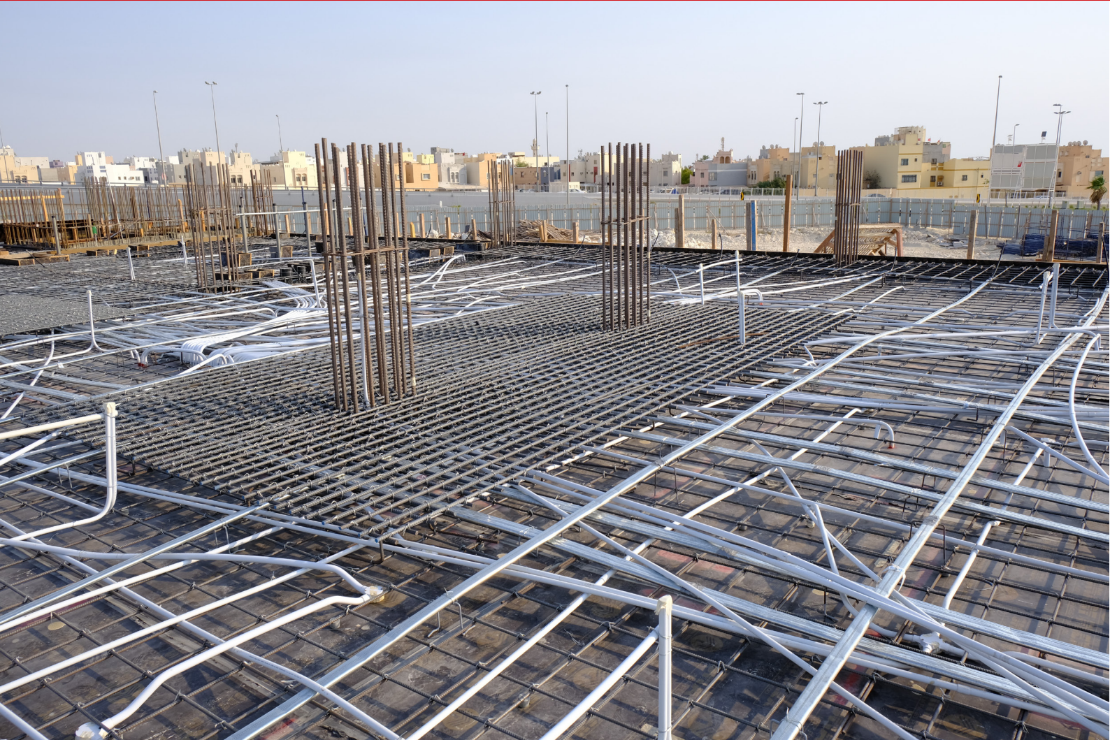
Figure 1: Cast-in conduits with junction boxes laid on slab
